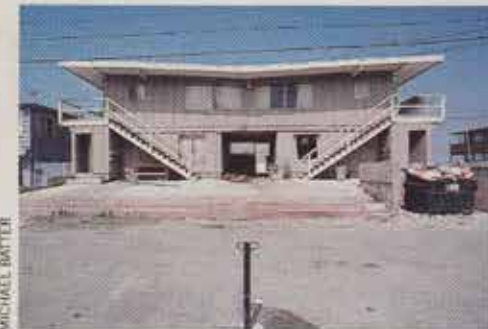
Batter Kay Associates, Inc. transformed the haggard, eight-unit, beachfront apartment building above into the sleek, International-style, five-unit condominium complex at the top of the page. In the process, they replaced the kidney-shaped pool with a secure central-entrance courtyard and five garages—a priceless commodity in Del Mar.
